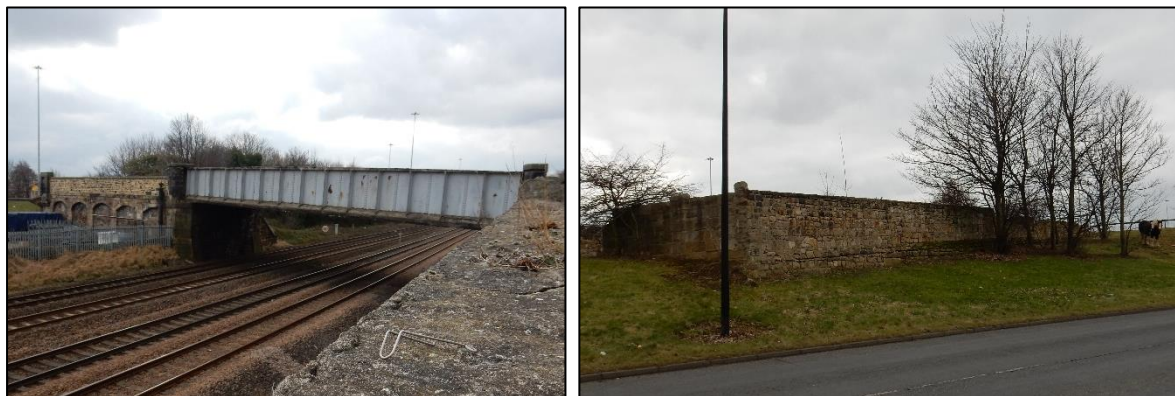
Plate 44. Left: Marsh Street Bridge with decorative supporting arches providing a ramp up to the bridge. Right: the remains of a late 19 th century building on the other end of Marsh Street Bridge
