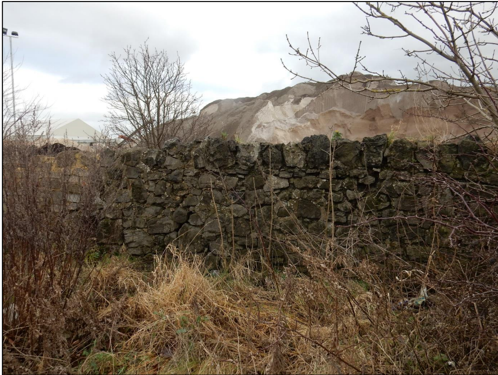
Plate 12. Boundary wall made of iron slag running along Forty Foot Road and the branch line.
