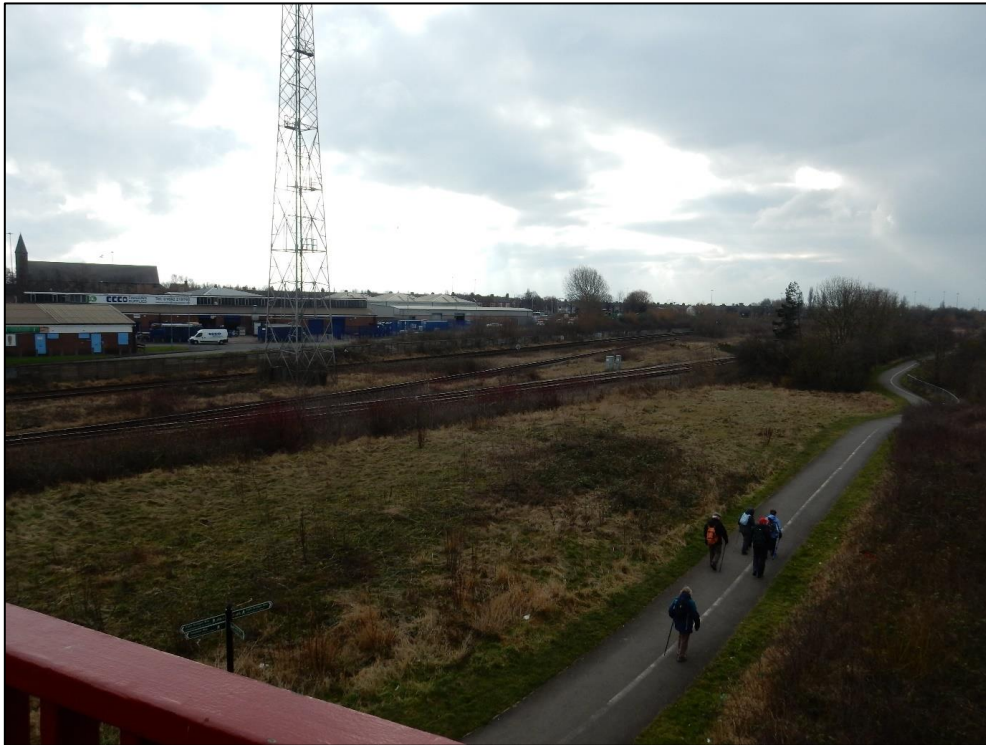
Plate 38. The shared cycle/footpath from Tees Newport Bridge looking SW with views of the trackbeds running alongside. This is also a junction with the Teesdale Way which leads straight to Middlesbrough and the Eight Bridges Way.
