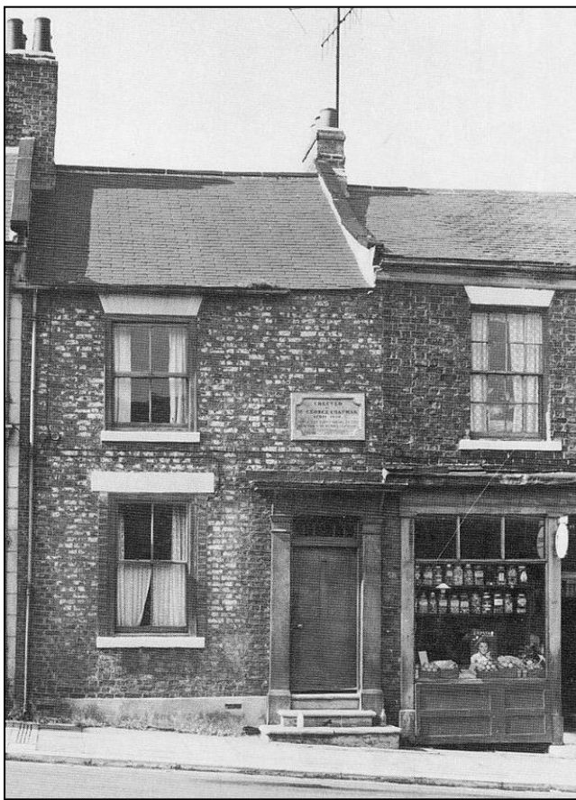
Plate 4. George Chapman's House on West Street (now demolished). The windows are Victorian replacements; the original windows would have been 8/8 sashes as seen on the first floor of the shop next door.
