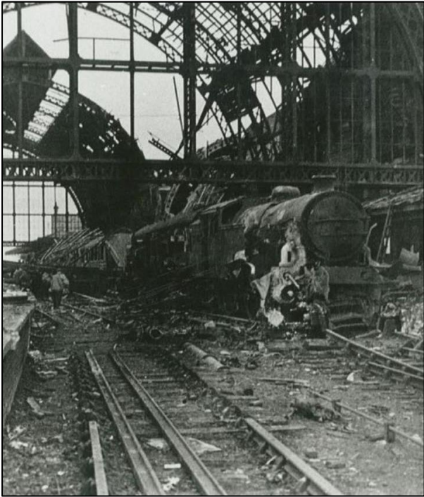
Plate 19. Bomb damage inside the sheds at Middlesbrough Station in the Second World War
