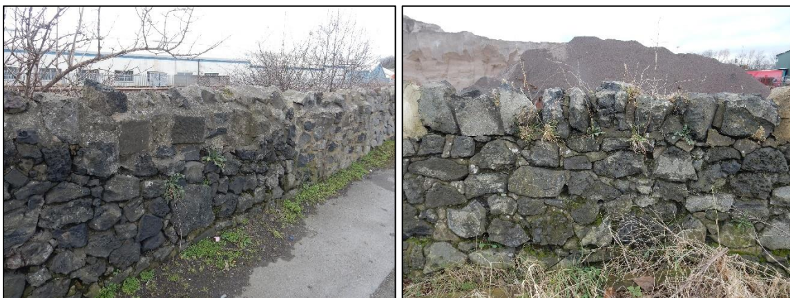
Plate 28. Boundary walls for the branch line on Riverside Park Road and Forty Foot Road. This iron industrial waste material must post date the second wave of expansion in Middlesbrough brought about by the discovery of iron ore in the Cleveland Hills in 1850. It has been patched up with various accessible materials and has become distinctive of the area. It is also of historic interest because it is associated with the iron industry. The walling on the right is opposite William Lane's Iron Foundry and perhaps originated from there in the 19 th century.
