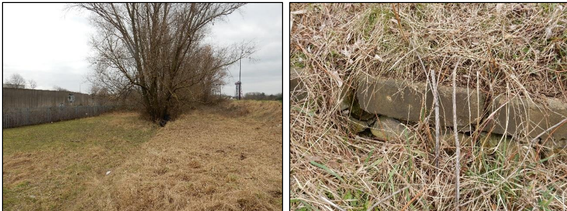
Plate 14. Remains of a disused trackbed running between the current trackbed and Riverside Park Road. This trackbed was a late 19 th century siding, but the low stone boundary walls and hedging are typical of early S&DR trackbeds.
