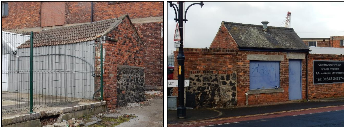
Plate 27. Two small buildings on Ferry Road which retain an early architectural character and surviving sections of iron slag walling
