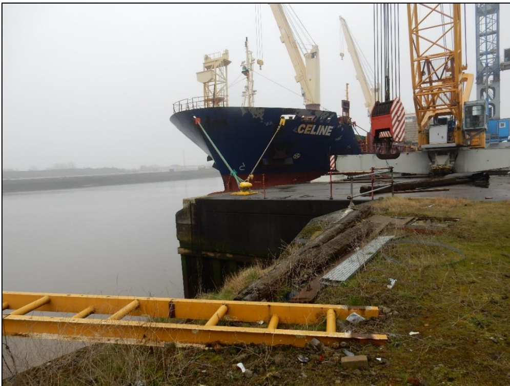
Plate 9. The extended quayside built by A. V. Dawson pushes the frontage further into the Tees, however to the NW the frontage is less extended and so the timberwork that survives there may be late 19 th century
