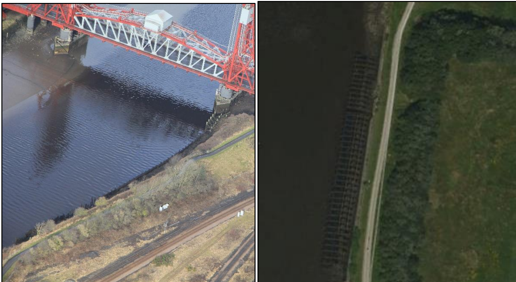
Plate 11. Left: Timber wharfs south of Newport Bridge. Right timber wharfs north of Newport Bridge. Both sets were being used in the 1930s
