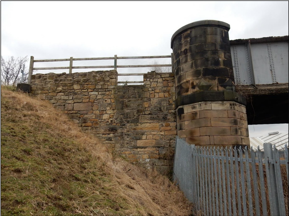
Plate 15. A late 19 th century railway bridge (Marsh Bridge or Fox Heads Bridge), now a footbridge, which sits over former sidings which once ran under this bridge (or an extended part to the north, since demolished). The walling on the left is the remains of a building with a window opening. The walls are made of reused dress sills or lintels from another structure. There was a signal box in this location in 1855 (OS 1 st ed 6 inch)
