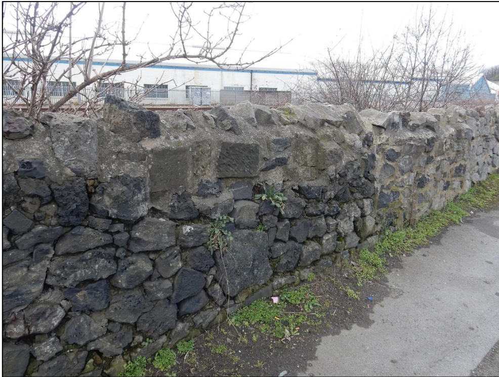
Plate 45. Boundary walls with the railway made of waste slag
